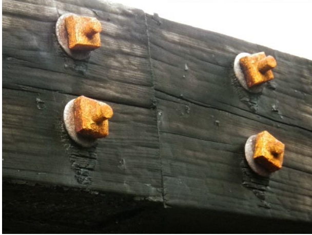
Bolts and charred support timbers
