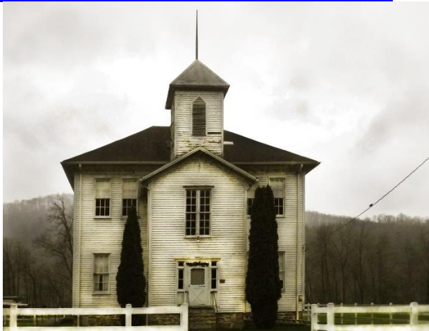
The unique clapboard building has a projected bay front & a square vented tower with a finial.
